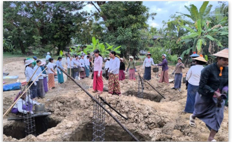
Construction of the Retreat Centre
